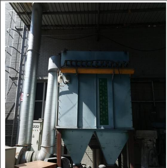
A photograph of a manual polishing waste gas treatment facility. It shows a blue industrial unit with a hopper, connected to silver metal pipes. The unit is located indoors or under a covered area.                                              |
