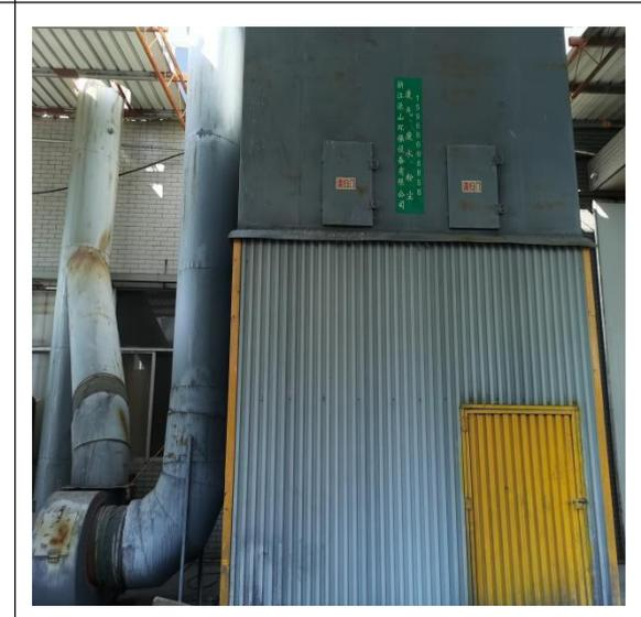
A photograph of an automatic polishing waste gas treatment facility. It shows a blue industrial unit with a hopper, connected to silver metal pipes. The unit is located outdoors near a brick building.                                          |
